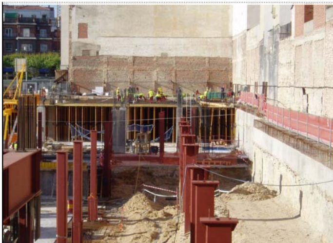
Excavation with partial slab support
