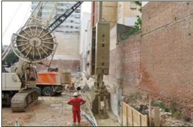
Diaphragm wall construction adjacent to an existing building
