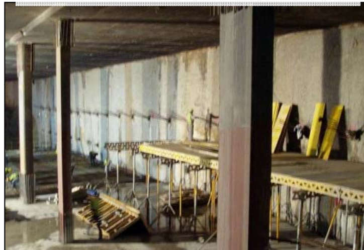
1800 kN ground anchors between floor slabs
