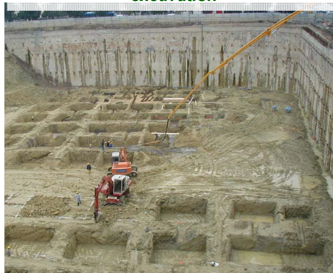
Footings and drainage blanket base excavation
