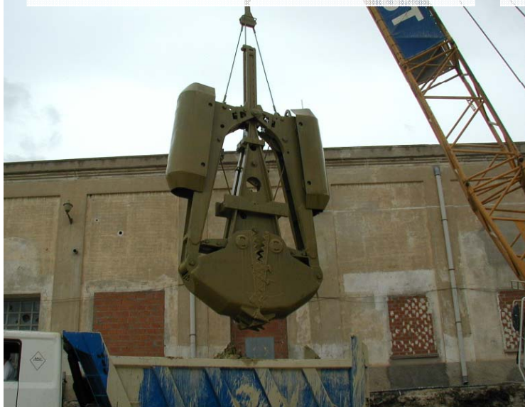
Diaphragm wall construction
